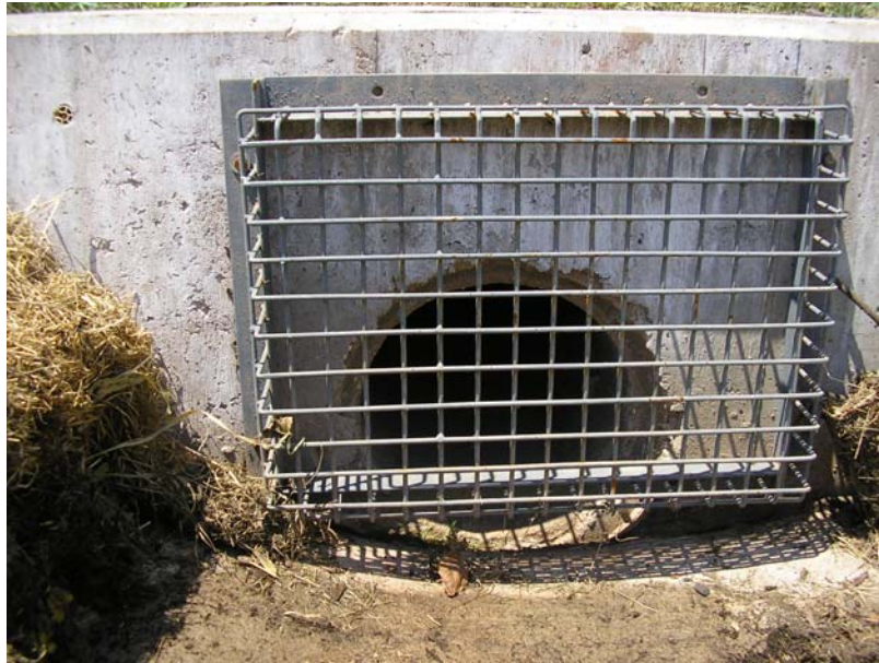
Outfall Structure at Basin at Colfax Road, large opening does not provide water quality
