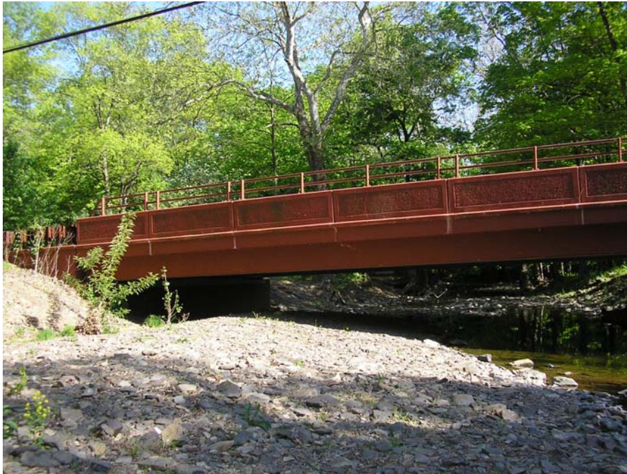
Bridge at Camp Meeting Avenue and Rock Brook, Four foot available between bridge and sediment deposits
