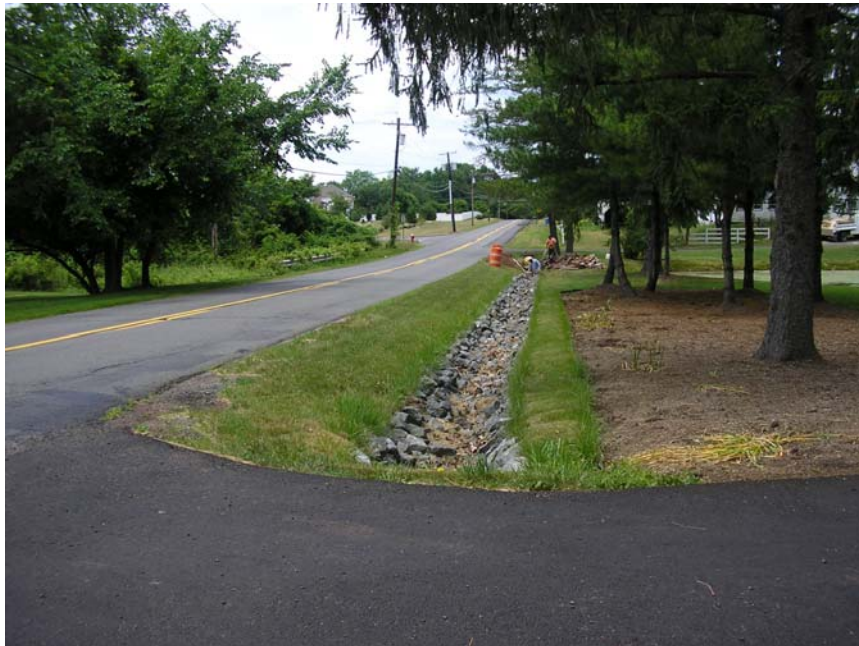
Swale repaired with rip rap, note gentle slope from pavement edge
